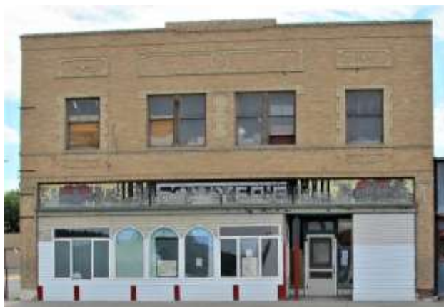
FIG. 9 - INCOMPATIBLE WINDOW TYPES & STYLES
